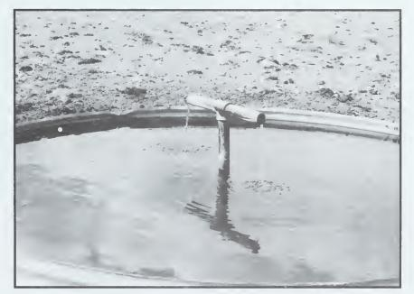
The same system is piped approximately 6 miles and serves four troughs that provide water to livestock from December 1 to April 15. In addition, small herds of deer and elk take advantage of the water sources.
